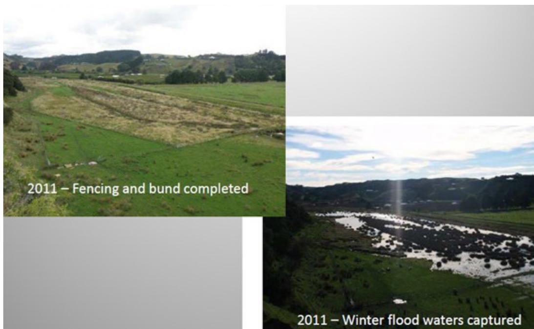
Figure 25. Phase 1 of the upper Ahuriri Estuary (Te Whanganui-a-Orotū) matuku-hūrepo habitat restoration showing the block before and after construction of the first bund to hold water within the wetland. *Photo: Hans Rook.*
